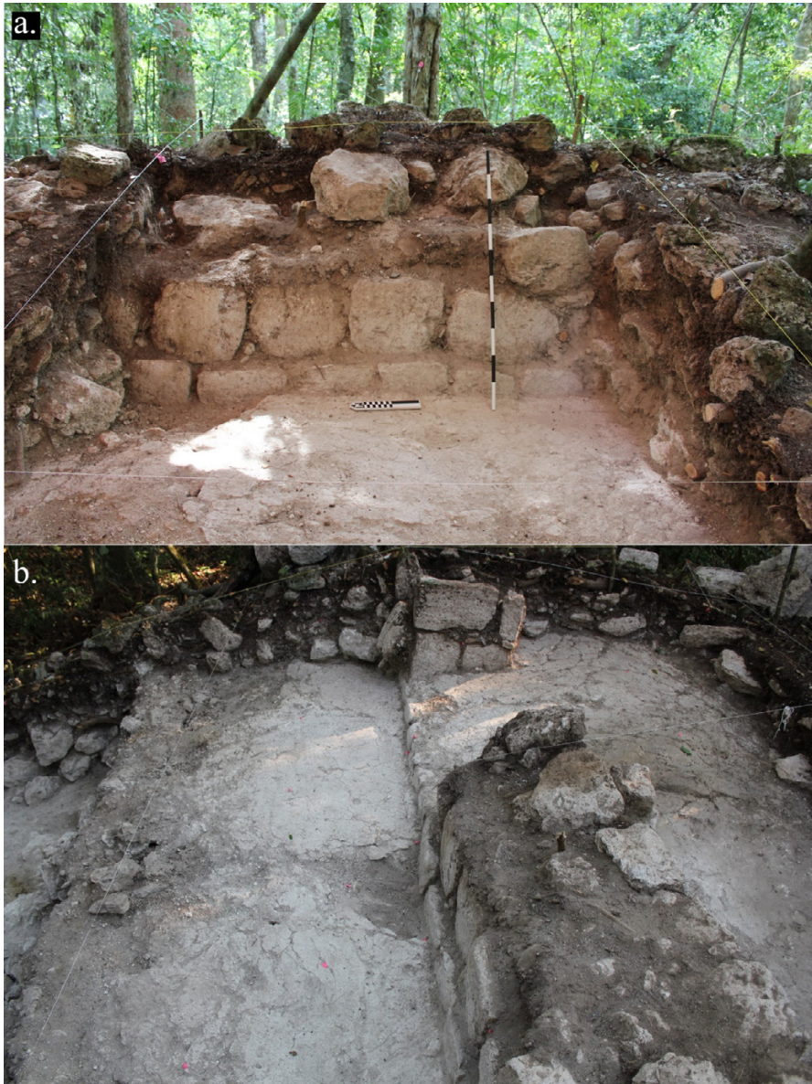
Figure 7. Ximbal Che, Structure 2, Terminal Architecture: (a) exposed portion of masonry wall of the superstructure, facing east; (b) terrace landing, showing possible cut through plaster and superstructure room. Photos by M.S. Longstaffe.
