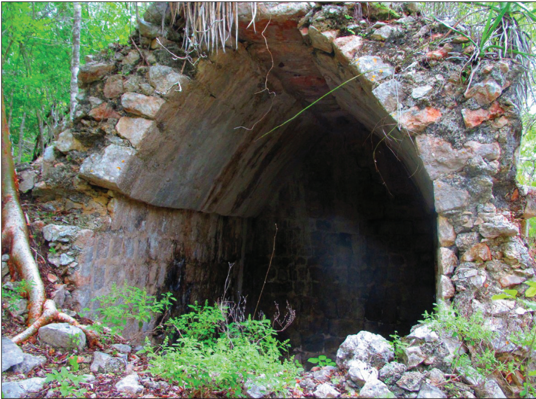
Figure 3. Photo of a partially collapsed vault at the site of Kiuic showing the amount of lime mortar that would have been necessary to construct these buildings (photo by author).
