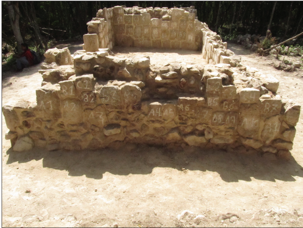
Figure 5. Western side of the principal vaulted masonry building in the northern group of Escalera Cielo. The lack of lower molding stones indicates that residents planned a future expansion of the structure but did not complete construction either due to lack of funds or because of the abandonment of the settlement.
