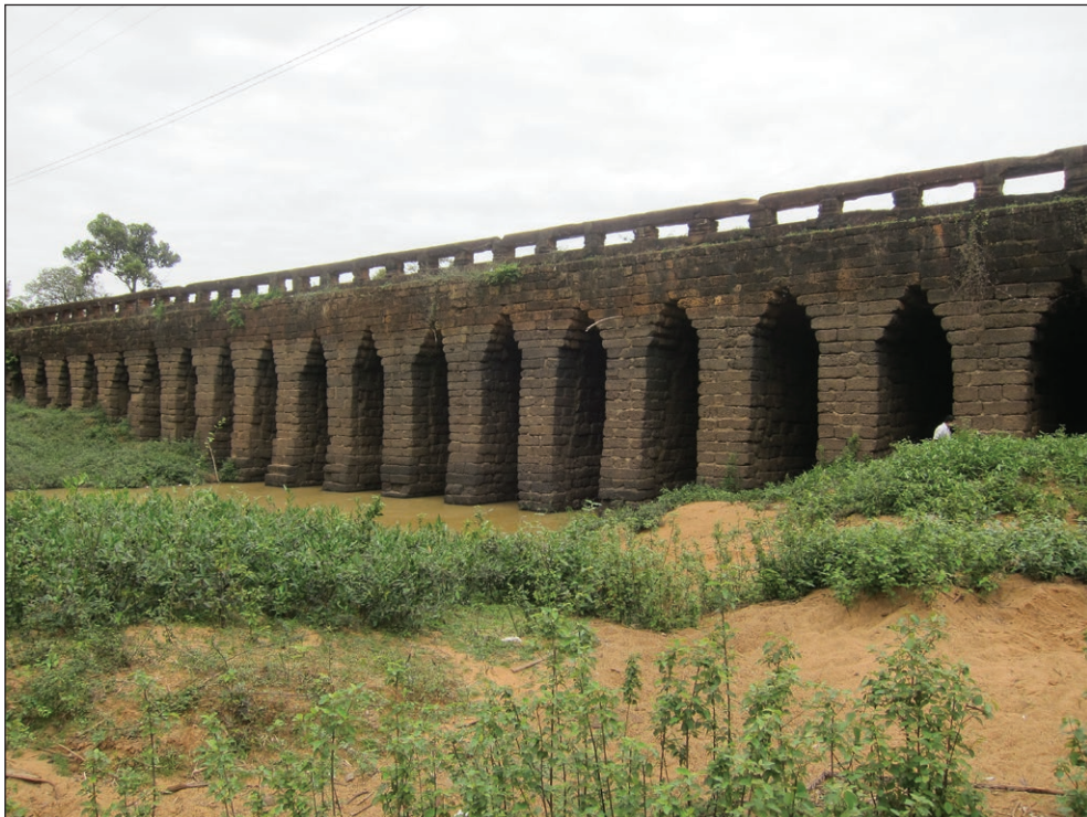
Figure 5. Spean Praptos Bridge, Cambodia.
